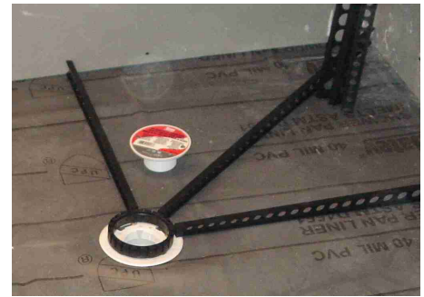
Quick Pitch installed with CURBSTILE
