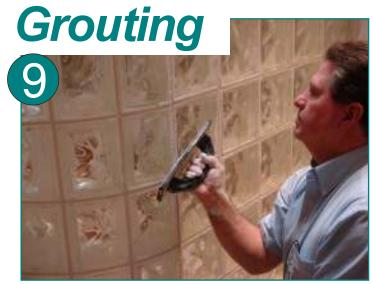
Follow instructions on grout bucket. Water measurement is crucial. Add water slowly. This grout resists the water at first and can become soupy if not careful. Let grout "slake" or sit in the bucket for at least 5 minutes (10 for colder job conditions) and then remix. This is critical for maximum grout strength. Apply grout to all seams except where the glass block meets wall and sill. Fill all voids and compact into seams of spacers with rubber grout float.
