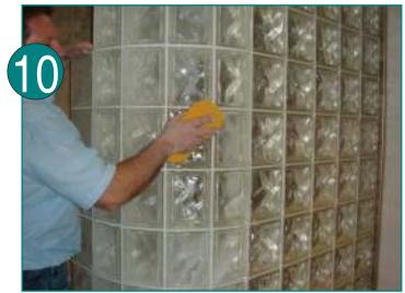
Use clean 45 degree water and wipe down block with a tile sponge. Wipe all joints and rinse after each pass ("clean swiping"). Rinse bucket and replace with clean water often. After this is done, wait 20 minutes to 1 hour depending on temperature, then repeat this process. Grout will start to cure and harden within 45-90 minutes depending on room temperature. After grout is dry, polish of haze with a clean rag.
