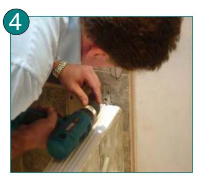
See that the panel is plum and level. Drive a screw through the upper hole in wall anchor. If attaching to marble or tile, predrill with a 5/32" masonry bit. Recheck panel. When perfectly plum drive in a second screw into lower hole.
