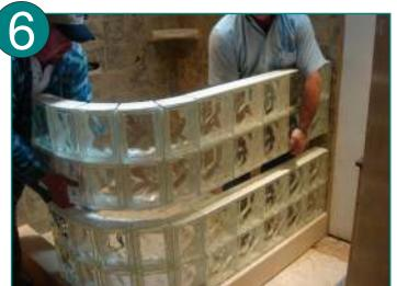
Place the second panel on top of the first. Push up to wall until vertical joints line up. Plum panel and attach panel anchor to wall. (Tip...If the panel is up against the anchor of the panel below it, and the joints don't line up; pry the lower panel away from the wall until they do.)
