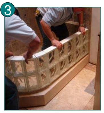
Set the first panel on the curb and push up to wall. Panel should be 1/8" from wall. (more if wall leans in at top).
