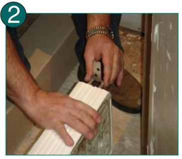
Apply a thick bead of silicone to center of sill and jam the height and length of panel.
