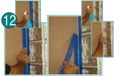
Spray the tooled joint again with a soapy water mixture (1 tbls dish soap to a full spray bottle of water) and smooth out the joint with your finger. When you have the desired finish, remove the tape, pulling it at a 45 degree angle. Once the tape has been removed, spray the joint and run your finger along it one more time to smooth out any imperfections from removing the tape. Repeat this process until all joints are sealed.
