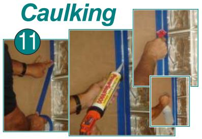
Make sure grout is completely dry. Wipe all dust from block, jamb, and sill. If there is any oil present, wipe with alcohol. Now apply blue masking tape to panel 1/8" from edge of glass. Also apply to wall and sill on both sides of panel. Apply sealant to perimeter, completing one side at a time. Spray tooling solution on joint (10% alcohol to water mixture). Using a Caulk Rite tool strike the joint, wiping the tool clean when sealant builds up on it.
