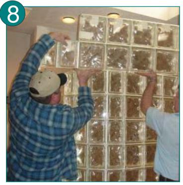
Because the top panel cannot be anchored it will rely on the silicone at the jam and between panels to hold it in place. Some top panels may need to be braced temporarily overnight to cure.
