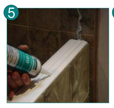
Apply a bead of silicone to the wall the height of the second panel. Apply two beads to top of spacer of first panel.
